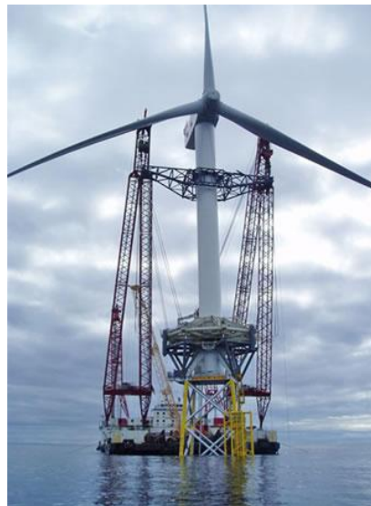
FIGURE 17: Setting up a wind turbine in an offshore wind farm
