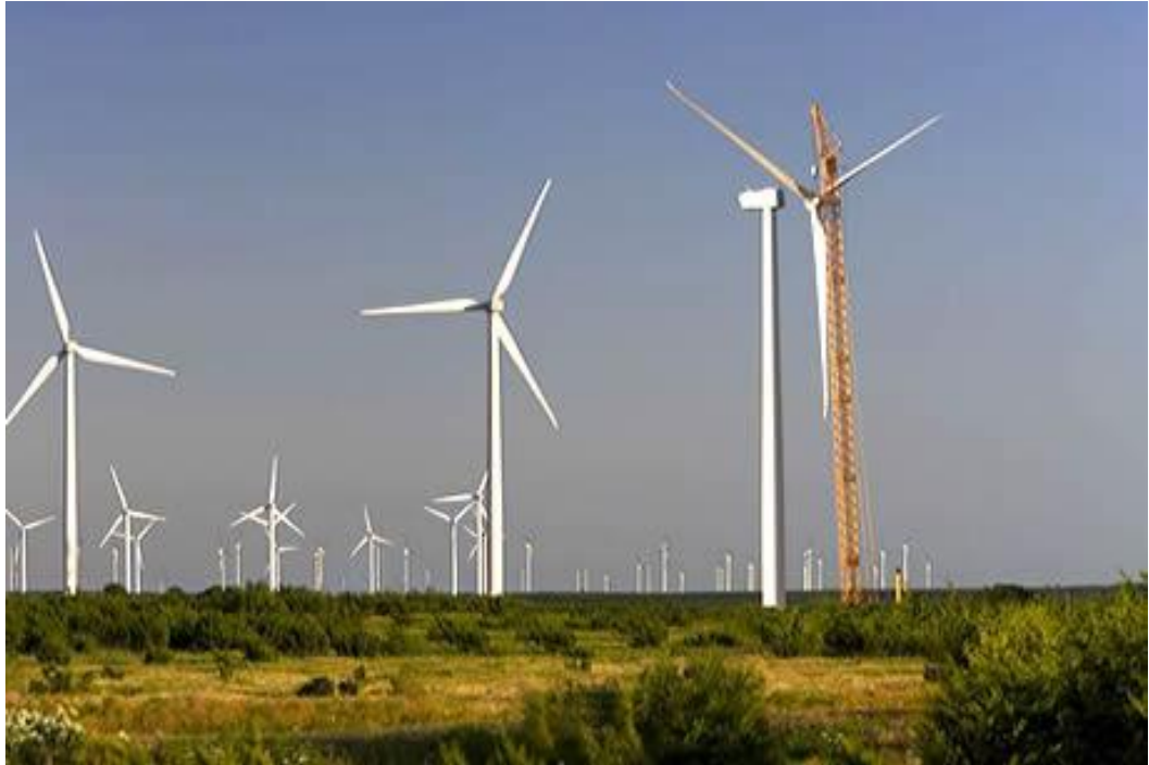
FIGURE 14: The largest wind farm in the world: Horse Hollow in Texas, USA. A wind farm equipped with 421 wind turbines that generate a total capacity of 735 MW (Wikipedia; House Energy 2010)
