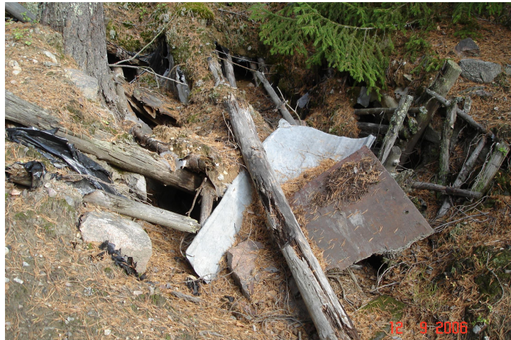
PICTURE 10. A collapsed structure near the top of the hill.
