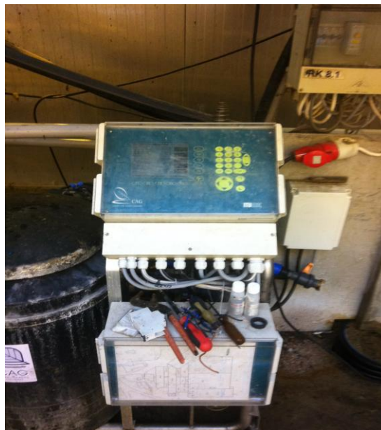
Picture 4 -Automatic Irrigating system
