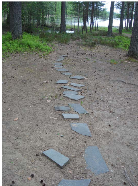
FIGURE 8: In the yard area, there could be better lightning and the risks for tripping should be minimized.
