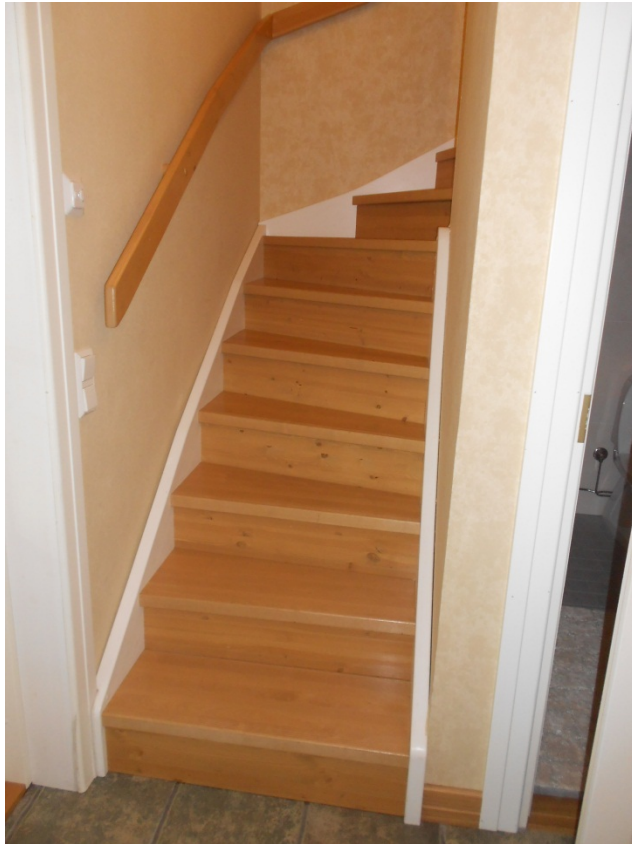
FIGURE 6: The staircase in Villa Hiidenmäki: Contrasts stripes would improve perception
